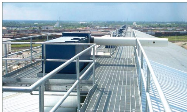
Figure 4. The FLSmidth distributive dust collection system significantly improved efficiency while reducing total power consumption by over 35%.
