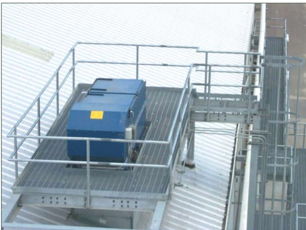
Figure 3. Operators are able to change filters via a top-access panel in the Donaldson Torit Dalamatric Collector.
