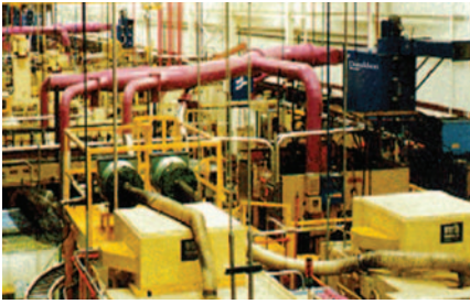
Fig. 2 — When installing a unit to collect fume from several welding stations, get the proper sized ductwork, collector, and fan.
