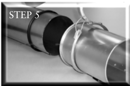
Cut piece of pipe put O-ring on cut pipe, slide nipple over
