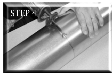
Drill access hole then cut with saw
